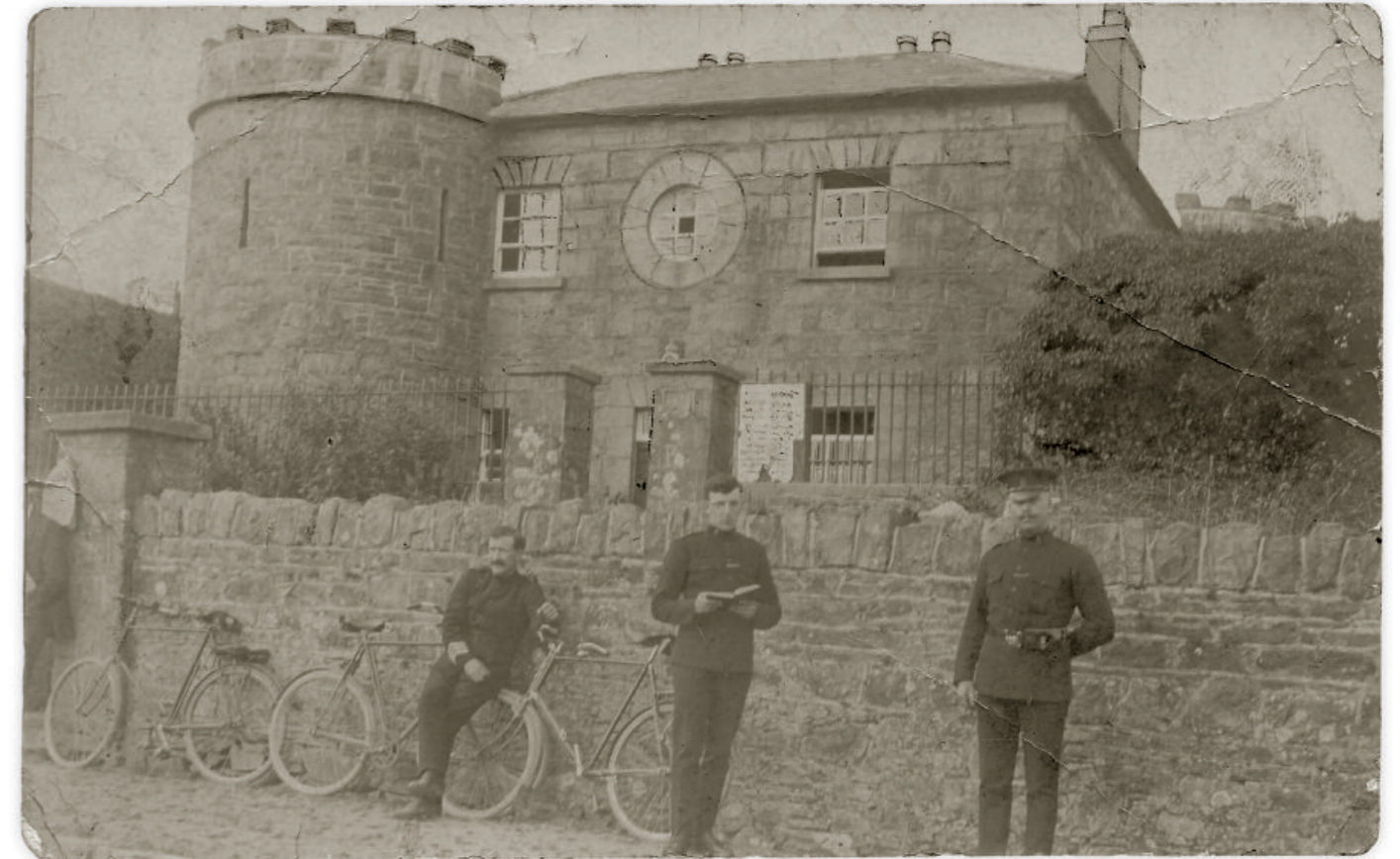
● Ballinamuck R.I.C. Barracks, County Longford (BMH/P2/001).
